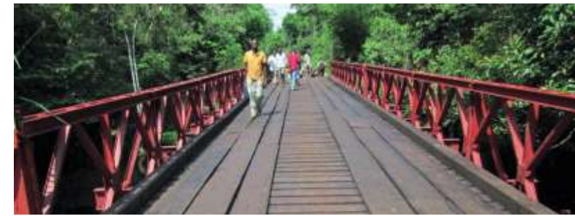
PROJECT: AGRICULTURAL SECTOR RECOVERY
