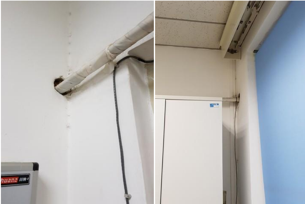
Figure 35 Example of Poorly Sealed Wall Puncture
