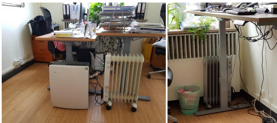
Figure 38 Personal Oil-Based Radiant Electrical Heater
