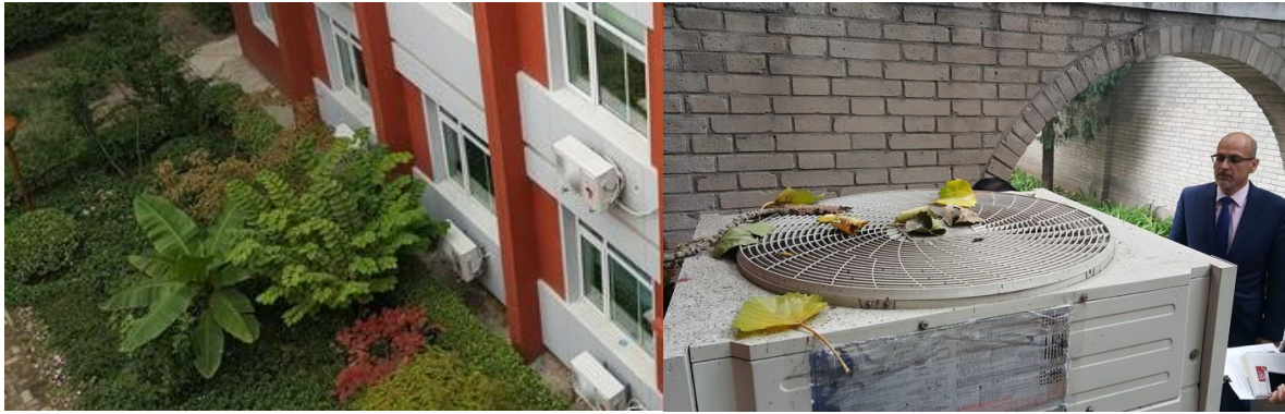
Figure 27 Air-Flow of Outdoor Units Obstructed by Plants and Leaves
