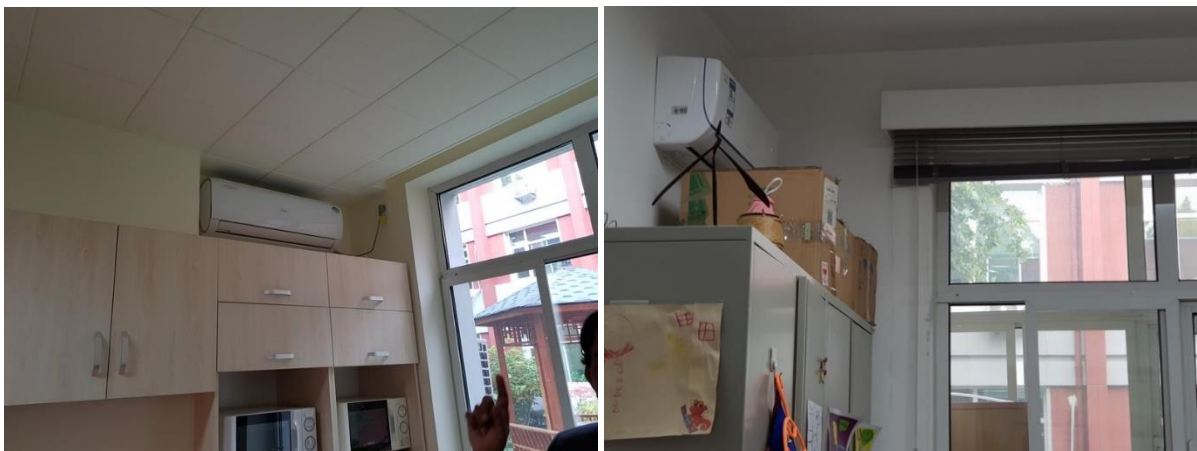
Figure 28 Obstruction of Air-Flow from Split-Units
