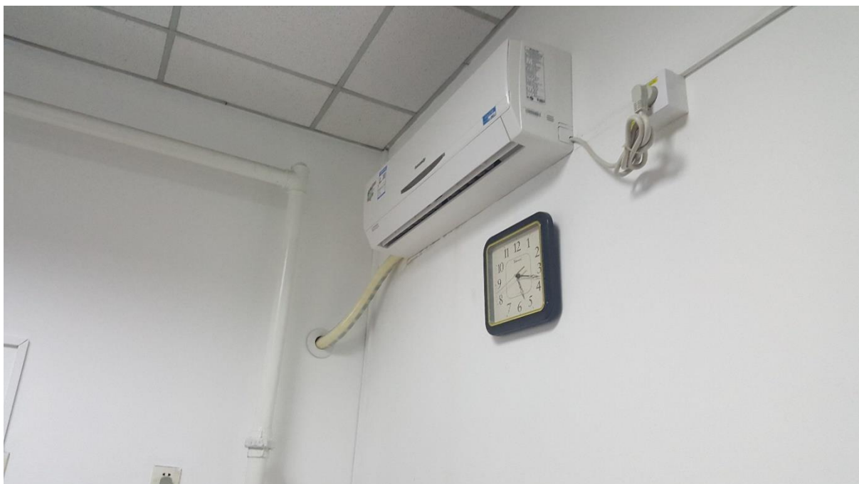
Figure 36 Well Sealed Wall Puncture
