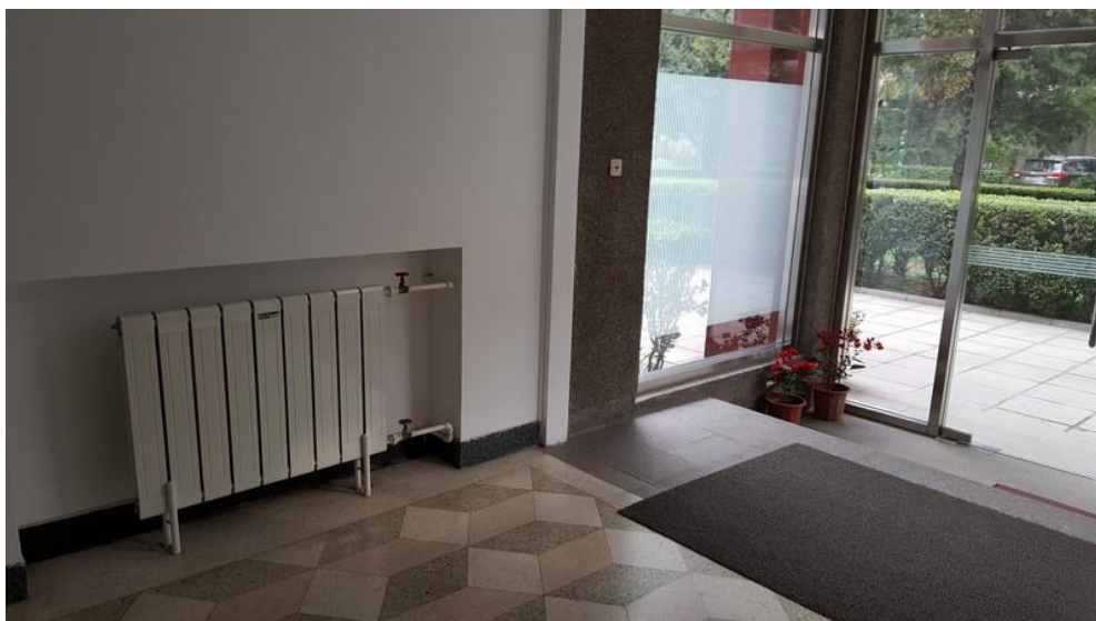
Figure 37 No Thermostat Control on the Radiator
