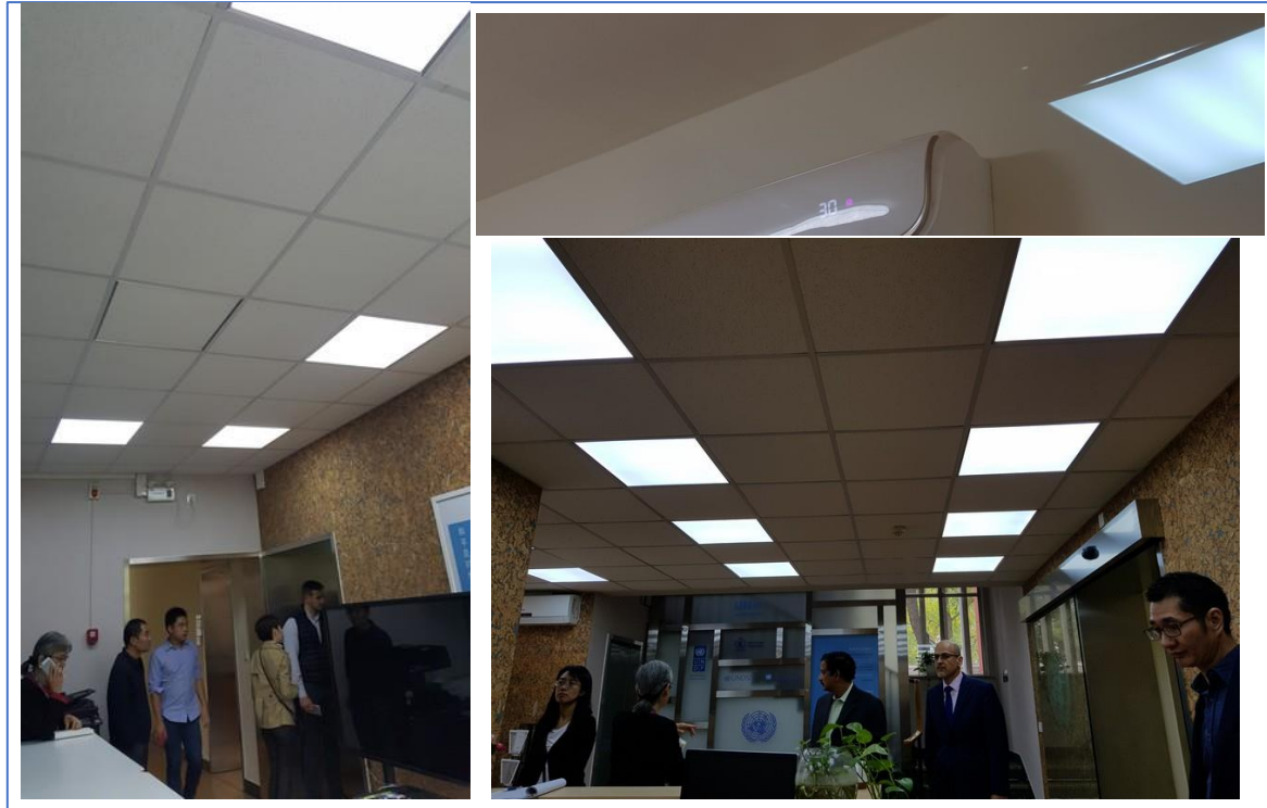
Figure 54 Panel Lights with Fluorescent/LED Lamps Inside
