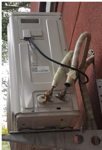
Figure 31 Poor Insulation of Refrigerant Piping
