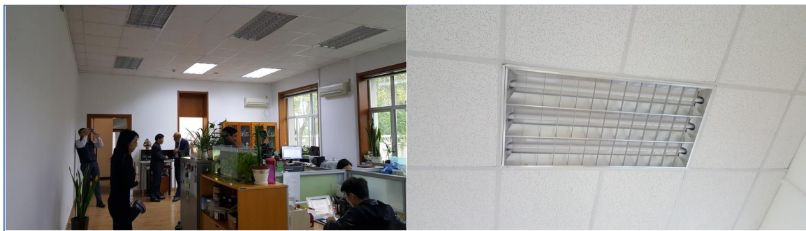
Figure 53 Fluorescent/LED Light Fittings for Offices
